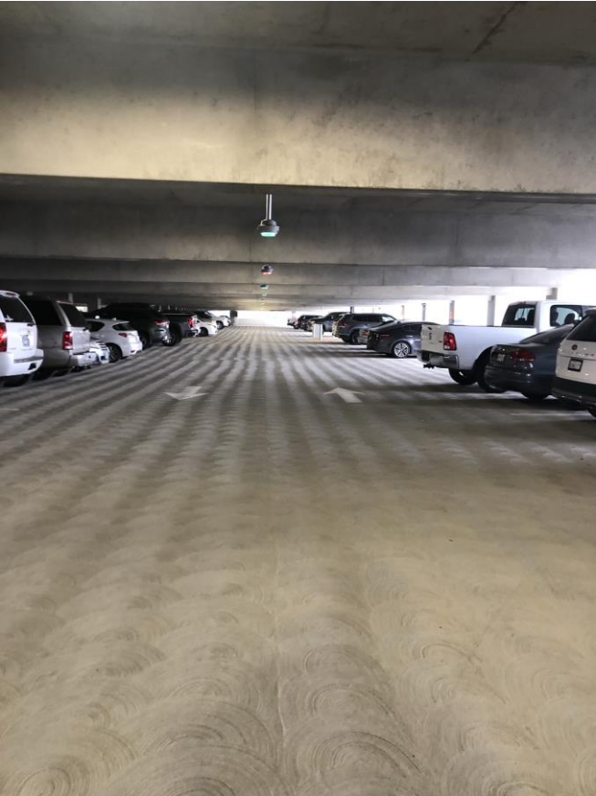
Airport Garage: Pre-embedded, camera-based sensors
