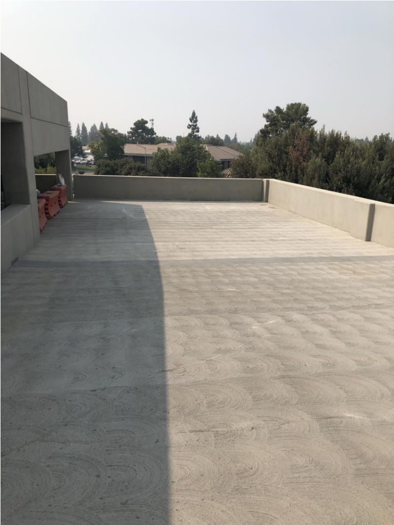
Airport Garage “WHERE ARE THE LOOPS?”
